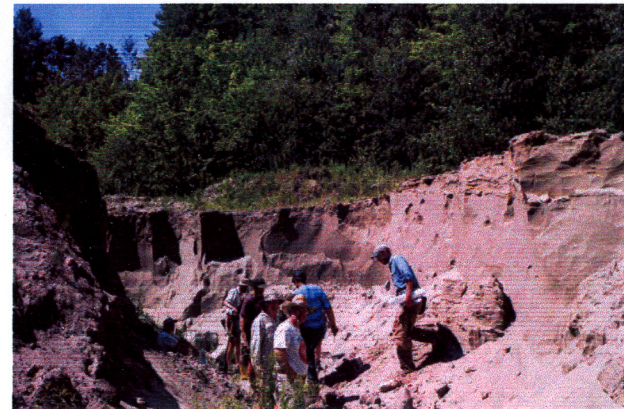
Stop #2: Up to 200 ft wide by 80 ft deep canyon eroded into ice-contact silty fine sands by an ephemeral tributary to the Great Brook. Erosion of this gully was initiated in the 1970s resulting from concentrated watershed, including channelization and removal of armor, contribute to the instability" which is associated with the absence of channel-spanning bedrock control [1]. This lower portion of the flow from agricultural runoff and lowering of the base level through active sand extraction. Fowler Pit, Plainfield, VT. (Photo: Jeff Hoffer)
