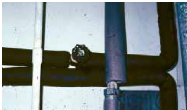
High temperature black insulation should be used on collector piping; gray insulation is OK for standard piping.
