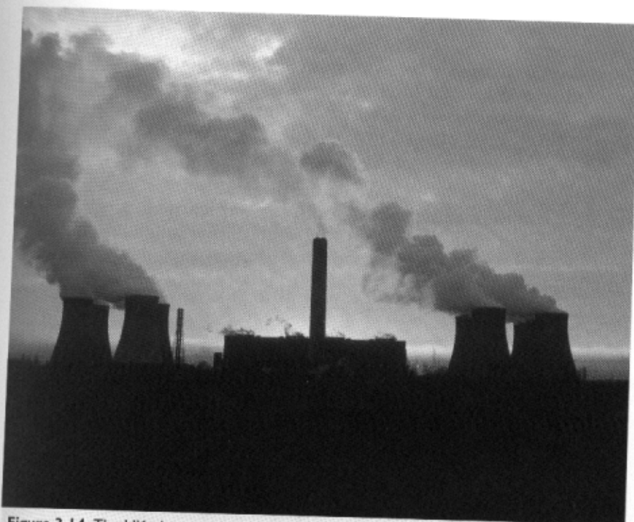
Figure 3.14 The UK electricity industry annually disposes of over 2 EJ of waste heat into the sky or the sea
