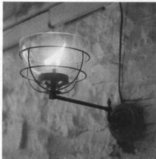
Figure 3.7 A naked gas flame is an extremely inefficient light source (an example in Judge's Lodgings Museum, Presteigne)
