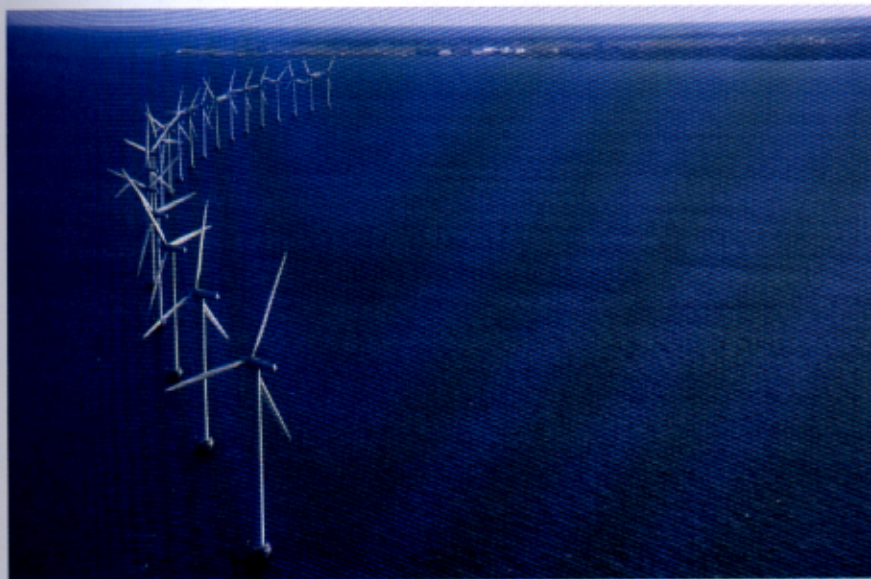
Figure 1.32 The Middelgrunden wind farm, completed in 2001, is located in the sea just off Copenhagen harbour in Denmark. It includes 20 two megawatt wind turbines, which provide 3% of the electricity consumption of the Copenhagen municipality
