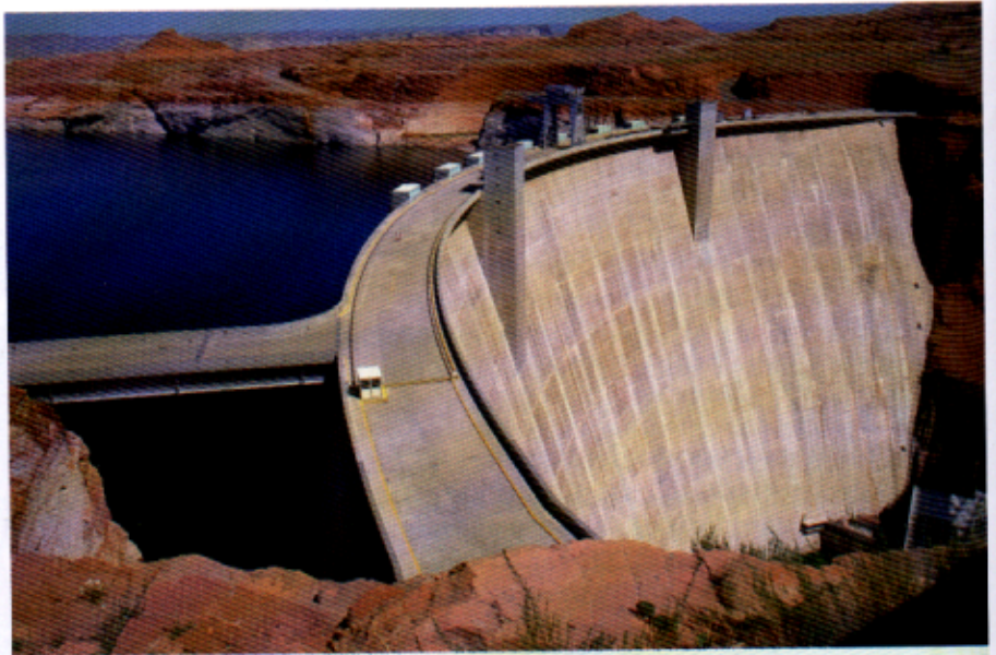
Figure 1.25 The large hydro-electric power plant at Glen Canyon Dam, Lake Powell, Arizona, which has an electrical generating capacity of 1300 MW. Lake Powell was formed with the construction of the Glen Canyon Dam in 1963, on the Colorado River in Page, Arizona. It is the second largest man-made lake in the United States and is 187 miles long
