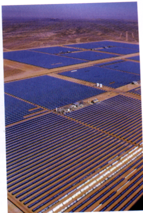
Figure 1.29 The largest 'solar thermal-electric' installation of its kind in the world, the Luz project in California's Mojave Desert, has a peak output of some 350 megawatts and occupies several square kilometres of land
