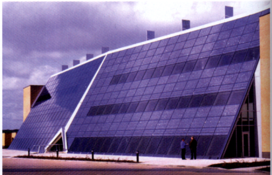
Figure 1.30 This 3500 m 2 solar office building at the Doxford International Business Park near Sunderland in the UK incorporates 646 m 2 of photovoltaic modules. These have a peak power output of 73 kW and generate some 55 000 kWh of electricity per year. The building is well insulated and uses passive solar design to maximise the use of natural daylight and to minimise space heating and air conditioning needs. It is also designed for natural ventilation and night-time cooling
