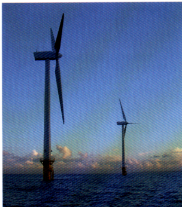
Figure 1.33 Britain's first offshore wind turbines, located 1 km away from the coast at Blyth harbour, Northumberland. The twin 2 MW turbines were installed in 2000 by a consortium including AMEC, Border Wind, Shell Renewables and the Dutch electricity utility Nuon
