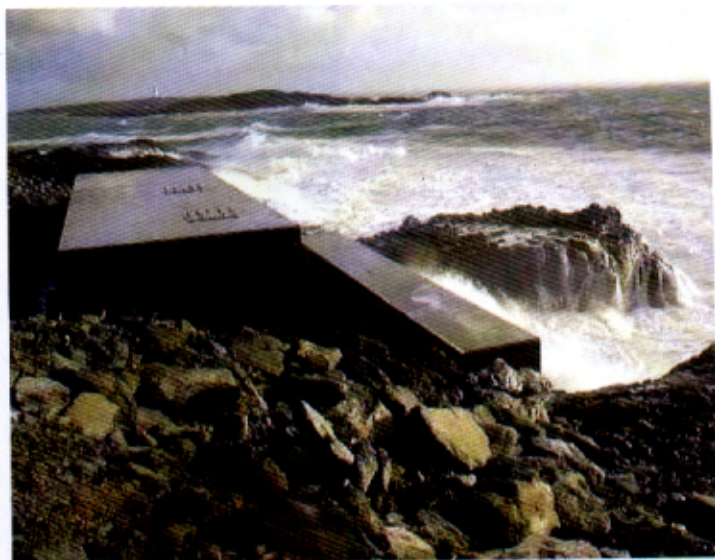
Figure 1.35 The 500 kW 'Limpet' wave energy plant installed in 2001 on the Scottish island of Islay
