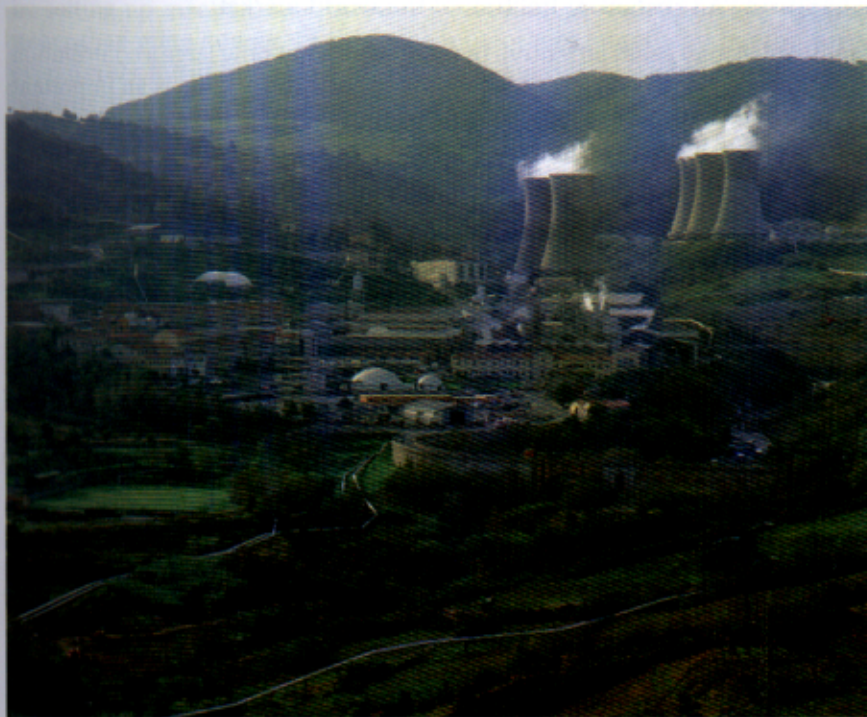
Figure 1.38 One of the geothermal power plants at Larderello, Italy, used to provide electricity and hot water
