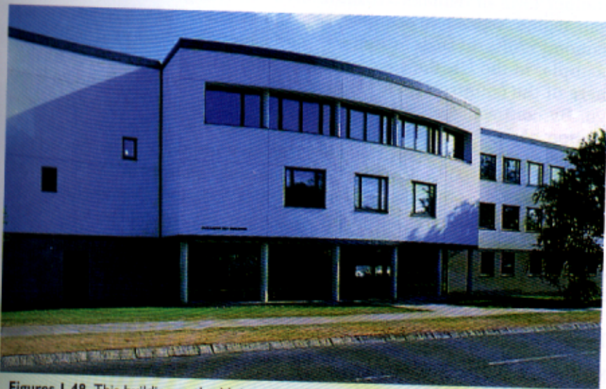
Figures 1.48 This building at the University of East Anglia consumes less than half the energy of a conventional air-conditioned building of comparable size and function
