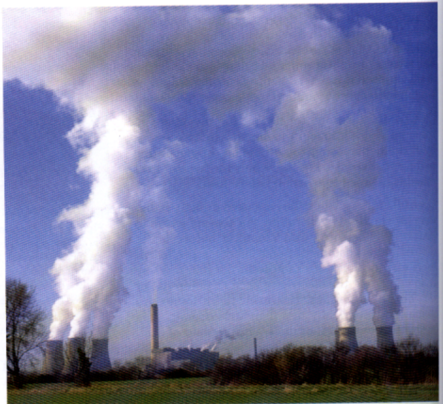
Figure 1.44 This coal fired power station at Didcot, Oxfordshire, UK, was commissioned in 1972 and has a capacity of 2000 MW. Two-thirds of the energy content of the fuel burned in such power stations is dissipated by the cooling towers to the atmosphere in the form of steam
