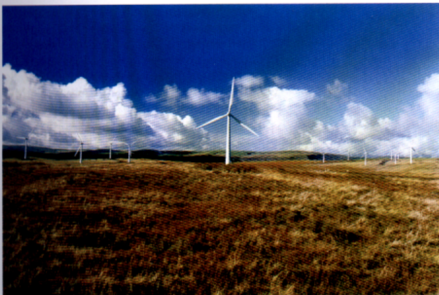
Figure 1.31 This wind farm, at Carno in mid-Wales, is one of the largest in Europe. It incorporates 56 wind turbines, each with a rotor diameter of 44 metres and a tower height of 31.5 metres. The total installed capacity is 33.6 MW, sufficient to provide power for some 25 000 homes
