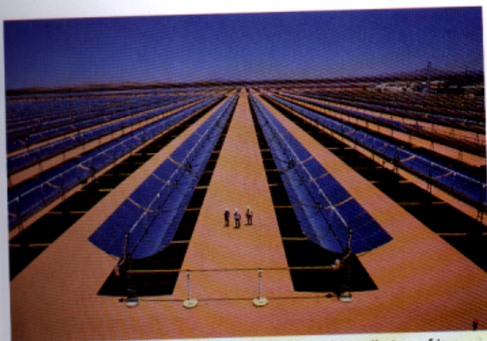
Figure 1.29 The largest 'solar thermal-electric' installation of its kind in the world, the Luz project in California's Mojave Desert, has a peak output of some 350 megawatts and occupies several square kilometres of land
