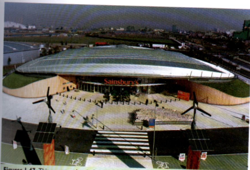
Figures 1.47 This supermarket in London is designed to use half the electricity of a conventional new food store of similar size
