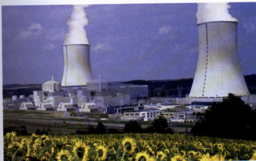
Figure I.20 The Civaux Pressurized Water (PWR) nuclear Reactor near Poitiers, Vienne, France. In 2000, France produced 77% of its electricity from nuclear power
