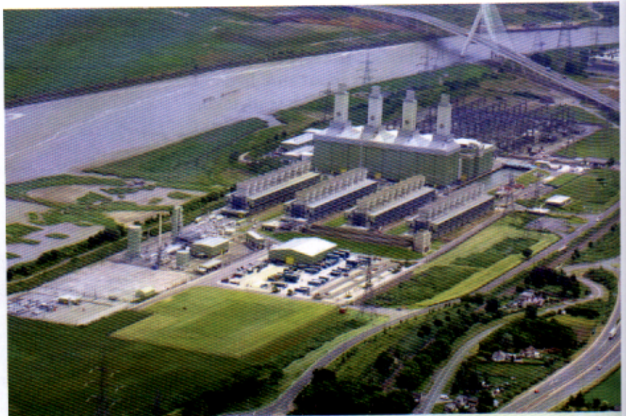
Figure 1.43 This combined-cycle gas turbine power station at Deeside in the UK was commissioned in 1994 and has an output of 500 MW
