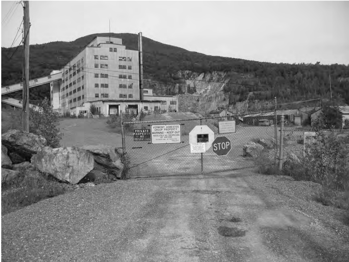
STOP 2a. VIEW OF MINE BUILDINGS AND THE LOWELL QUARRY BEYOND.
