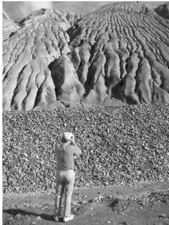
STOP 2c EROSION GULLIES ON TAILINGS PILES
