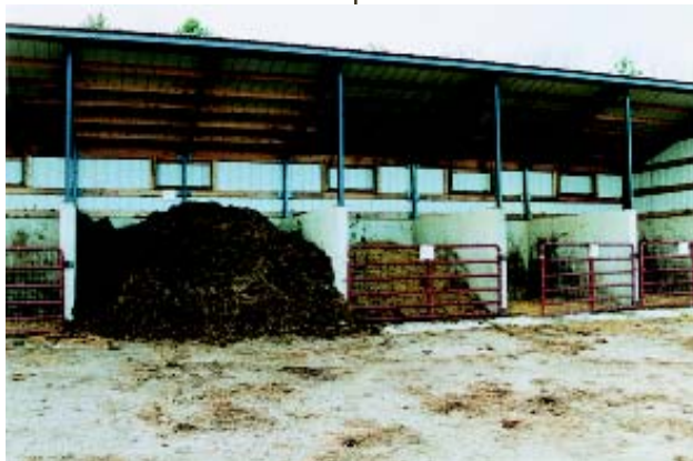
Multiple bin composting structure; note gates on fronts of bins.
