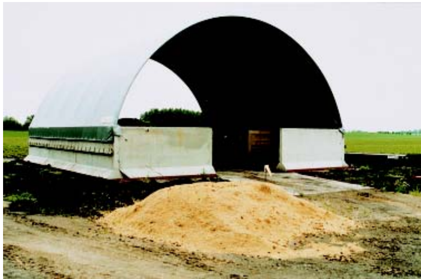
Hoop structure with six bins; note concrete apron and sawdust pile in foreground.
