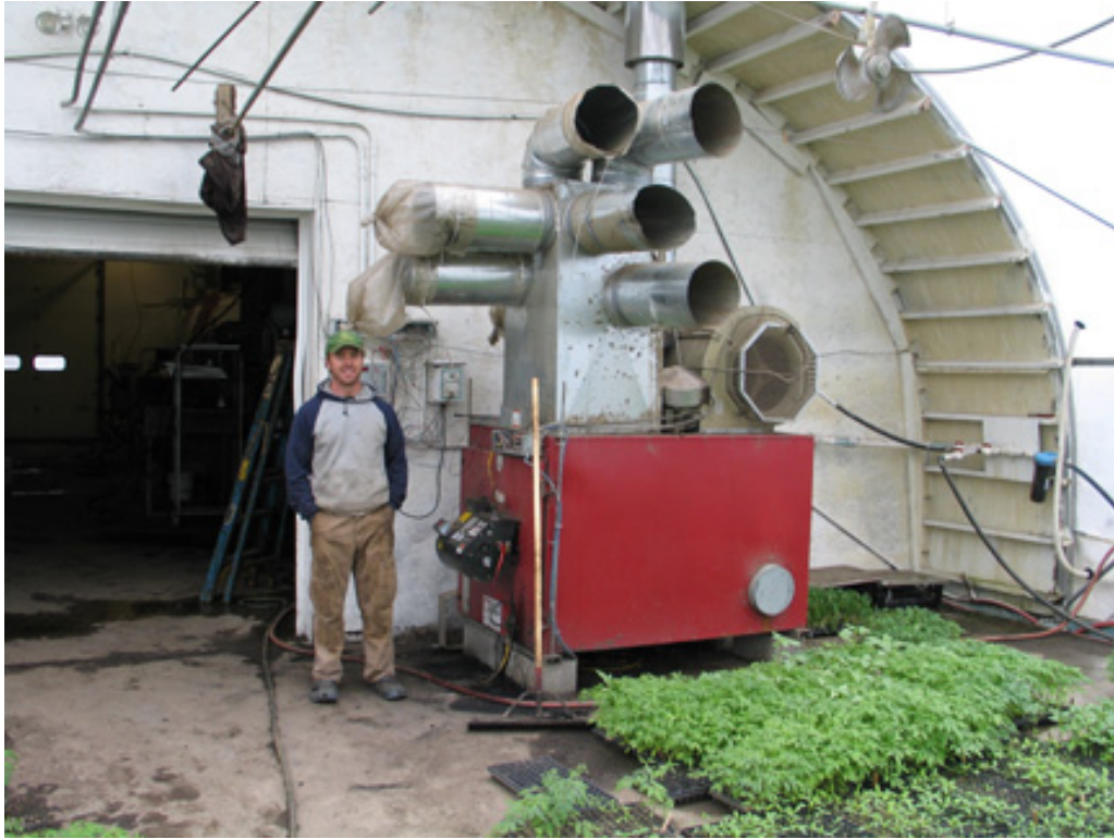
Figure 29 - Pete Johnson, Pete's Greens (Craftsbury) with Clean Burn 500, waste vegetable oil furnace.
