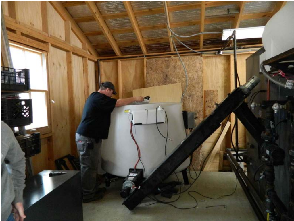
Figure 33 - Jason Martin, Woods Market Garden (Brandon) checks the fuel feed in the day bin.
