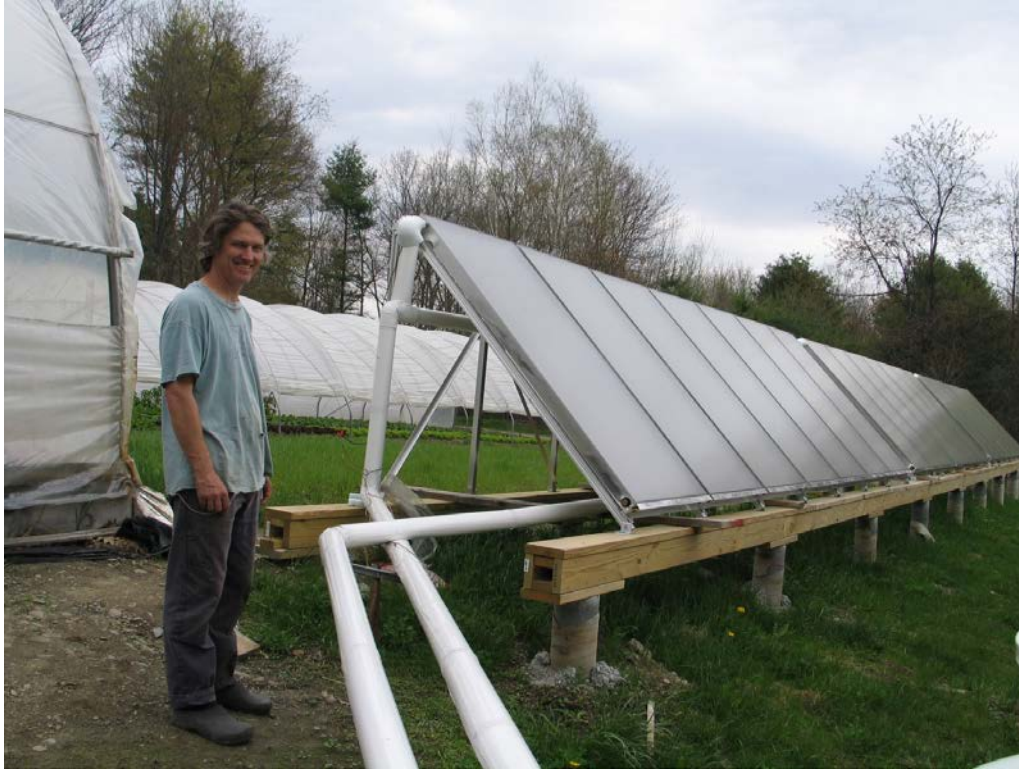
Figure 28 - Mike Collins, Old Athens Farm (Putney) stands next to his flat panel solar hot water heating system. While not biomass, solar is an alternative heating source that growers often ask about and this project was intended to generate real-life data for assessing the feasibility of solar to heat greenhouses in our region. In this case the solar system was tied into a small scale wood biomass boiler to heat hot water for the greenhouse and the farmer's residence in the off-season.
