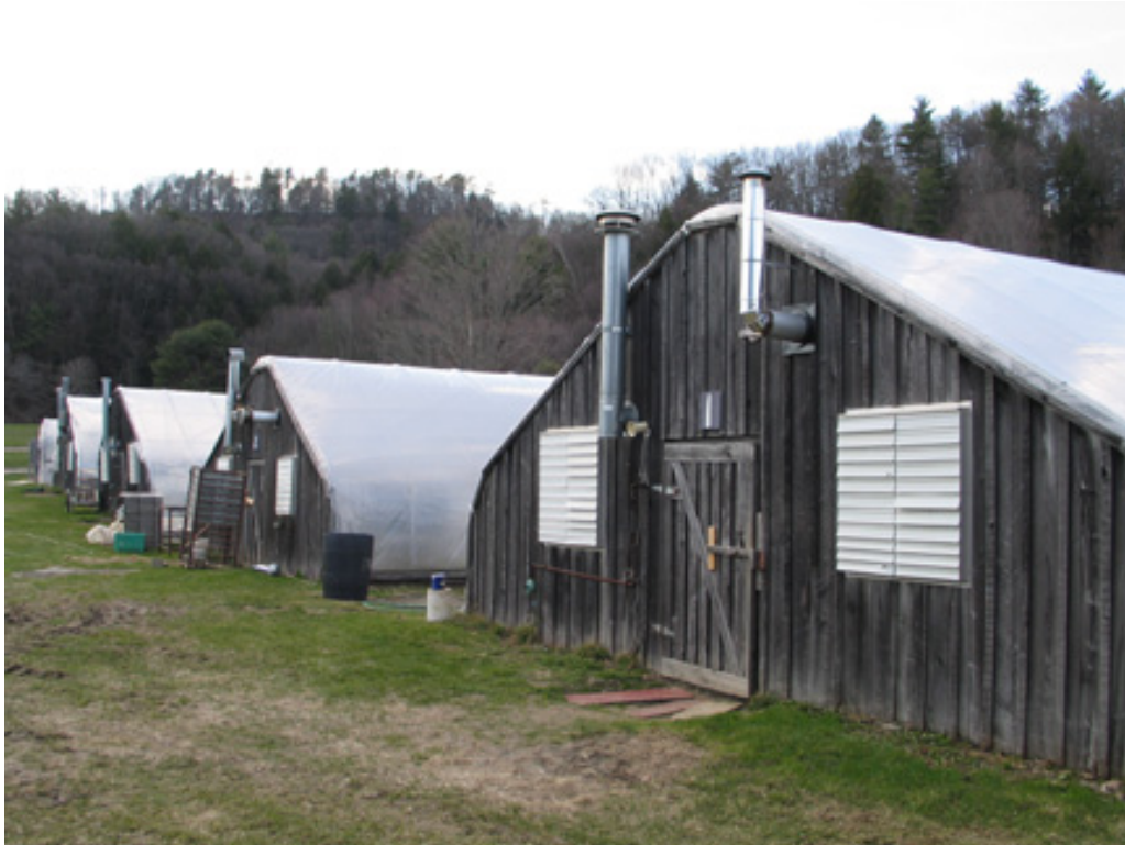
Figure 14 - Two chimneys on this greenhouse at Harlow Farm (Westminster); one is for the original propane heater and one is for the new LDJ biomass furnace.
