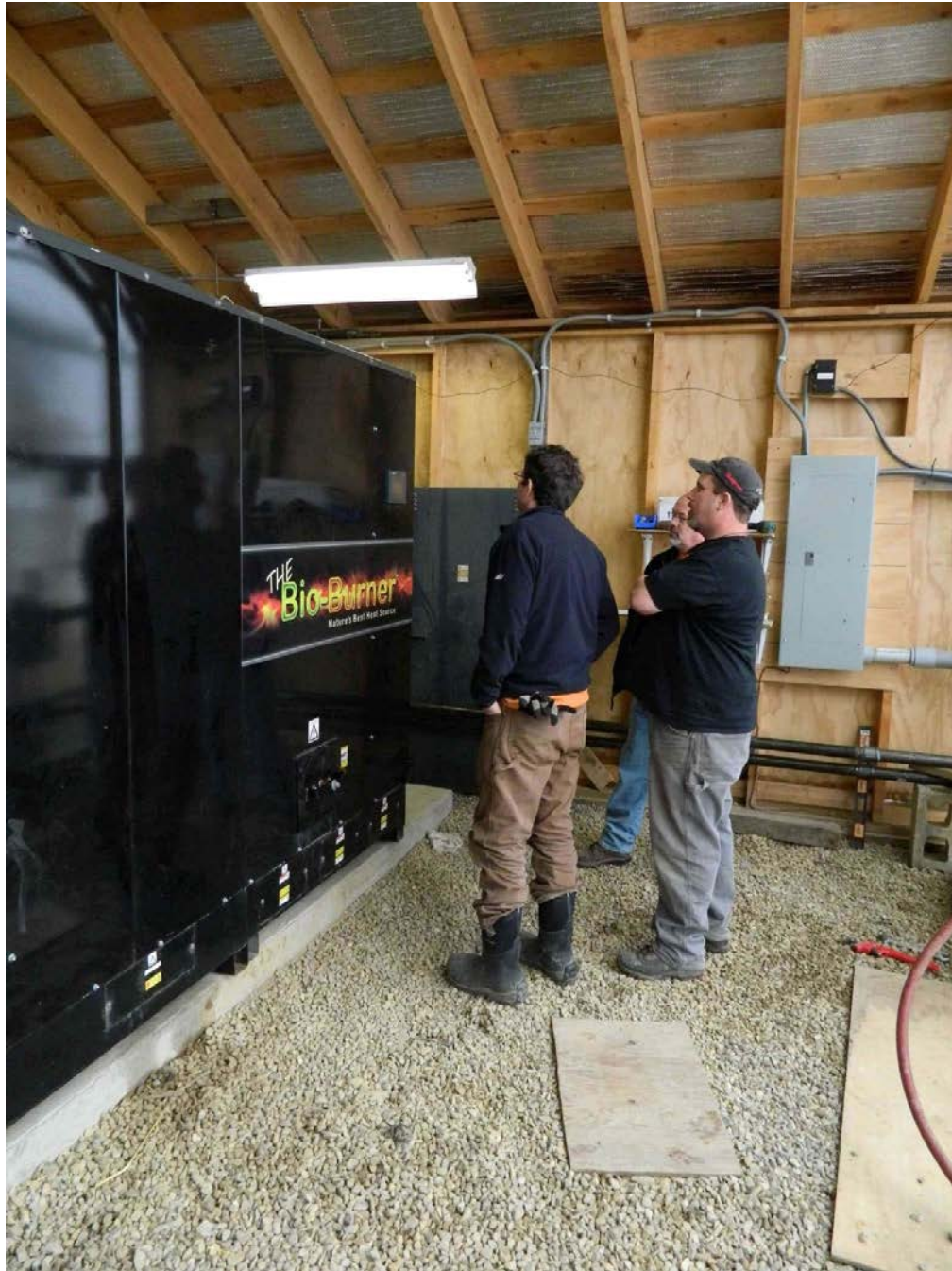
Figure 34 - John Satz (Wood's), Jason Martin (Wood's) and Scott Laskowski (LEI Products) go through boiler settings during the first startup at Woods Market Garden (Brandon).
