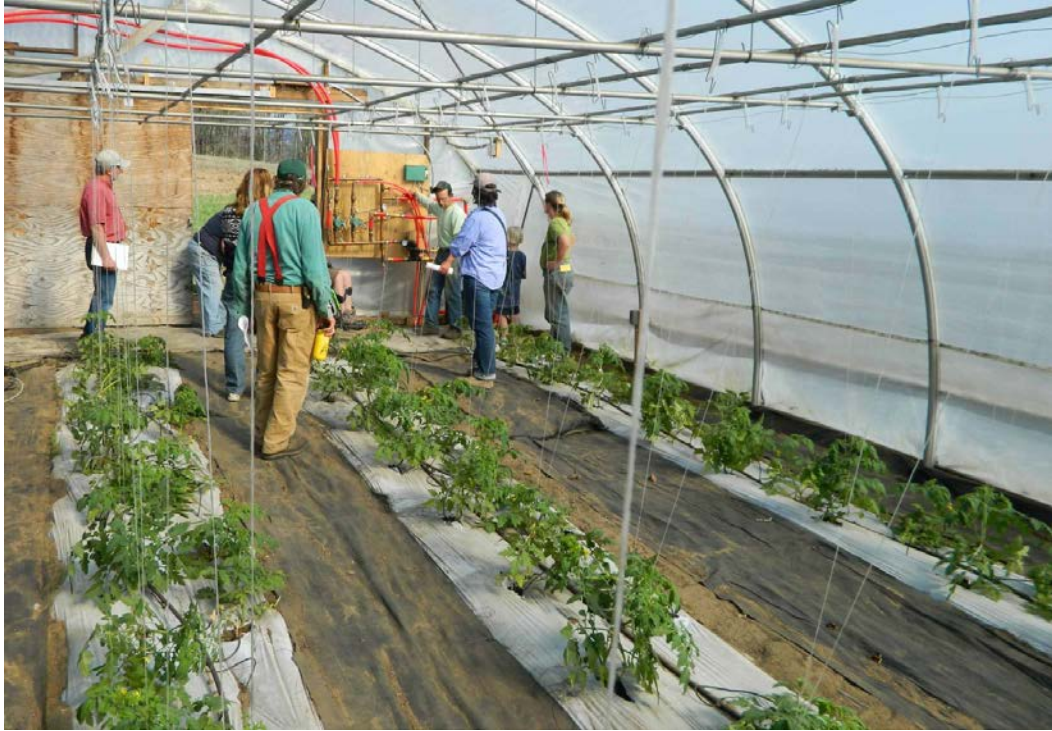
Figure 22 - Dave Marchant (Fairfax) shows the manifold for distributing hot water from the Maxim 250 boiler to both ground heat (under tomatoes in foreground) and to the greenhouse next door.
