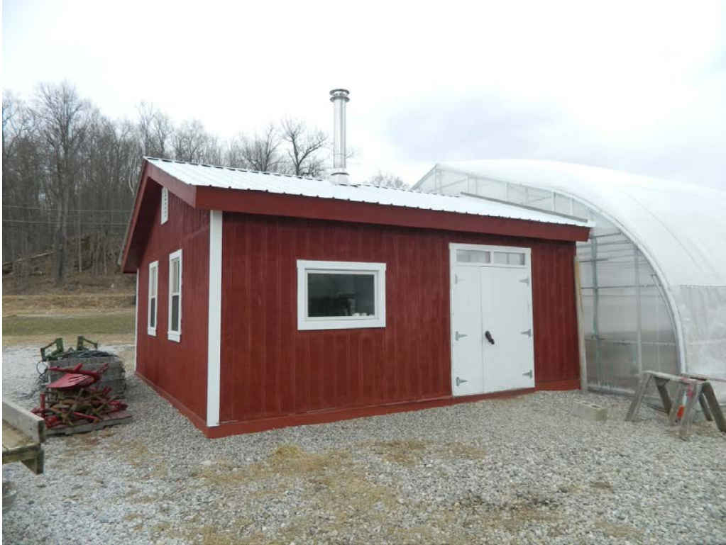
Figure 32 - Boiler House at Wood's Market Garden (Brandon).
