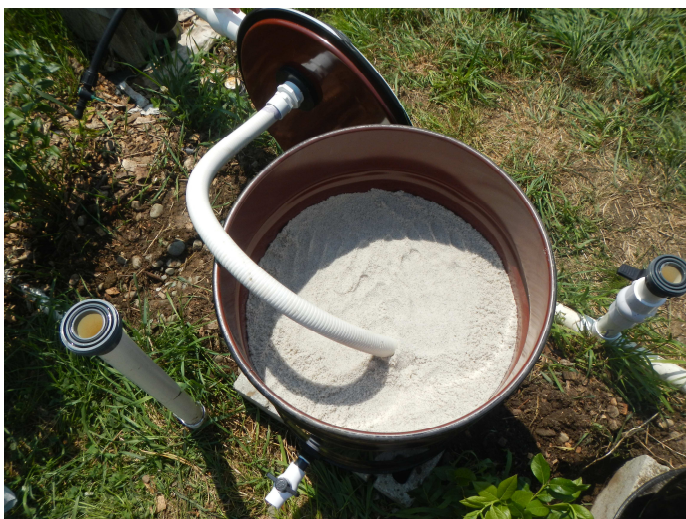
Figure 6. Filter sand placed in barrel.
