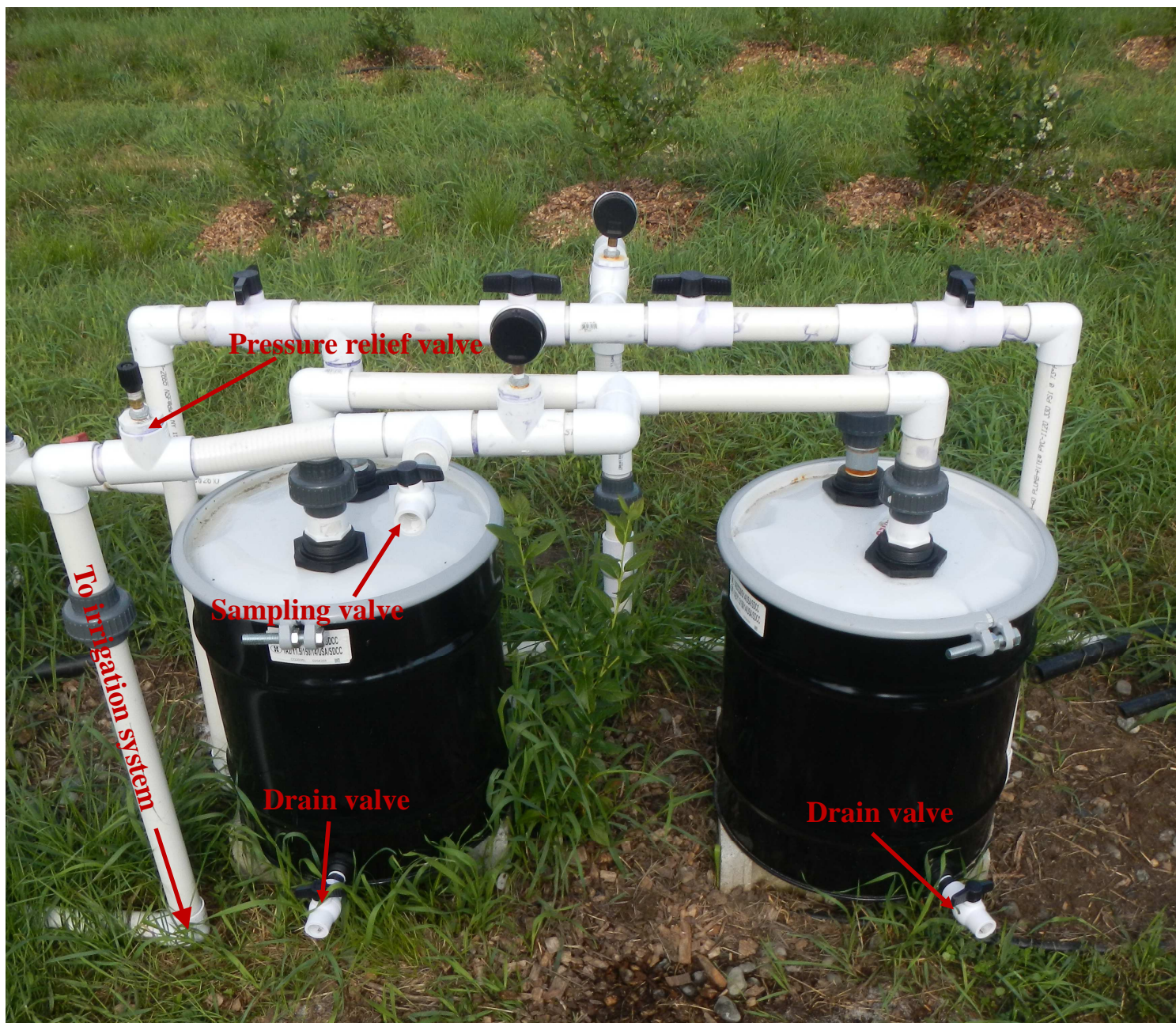
Figure 8. Rear view of sand filter system with various components identified. Note: Sampling valve and pressure relief valves were for evaluation only, they are not required if appropriate limit valve is installed.
