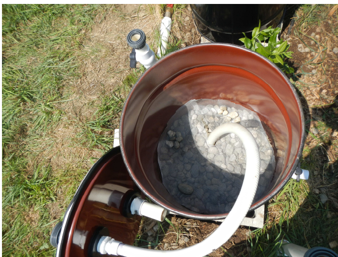
Figure 5. Clean gravel and screen over diffuser.
