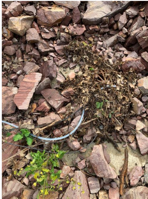
Figure 51. Beehive trash rack at the inlet of Kennedy Drive, hidden under debris from the incoming swale, running along Kennedy Drive.
