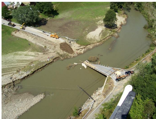
Photograph of Bridge 19 in Rochester, VT after Tropical Storm Irene. (VT Department of Transportation, 2011)
