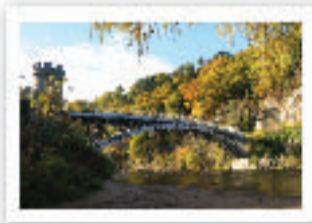
In 1812, after Telford designed Craigellachie Bridge - Scotland's first cast iron bridge - he took local advice and fortunately, built it five feet higher than planned
